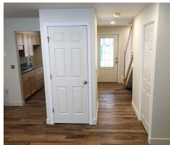
Sachem apartment entry AFTER renovation
