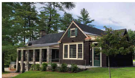
Renovations to the DOC House were completed in June. This project was led by Project Manager Jason Rouillard.
