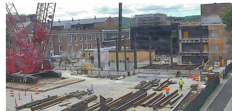
A large crane places vertical steel beams at the Irving Institute.
